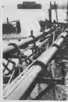
ONCE THE DYKES had been closed the flood waters were returned to the North Sea by means of an extensive network of pipes and powerful pumps. The small vessels in the center hold the pumps that suck water. UNA VEZ e dijknan a worde cerra e awa a worde deshali den Noordzee pa medio di un red extensivo di tubo y pompnan potentes. E barconan chikito den centro ta contene e pompnan cu ta chupa awa di dia y anochi.
